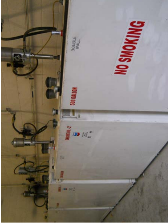
Figure 10 – Oil ASTs inside Garage
