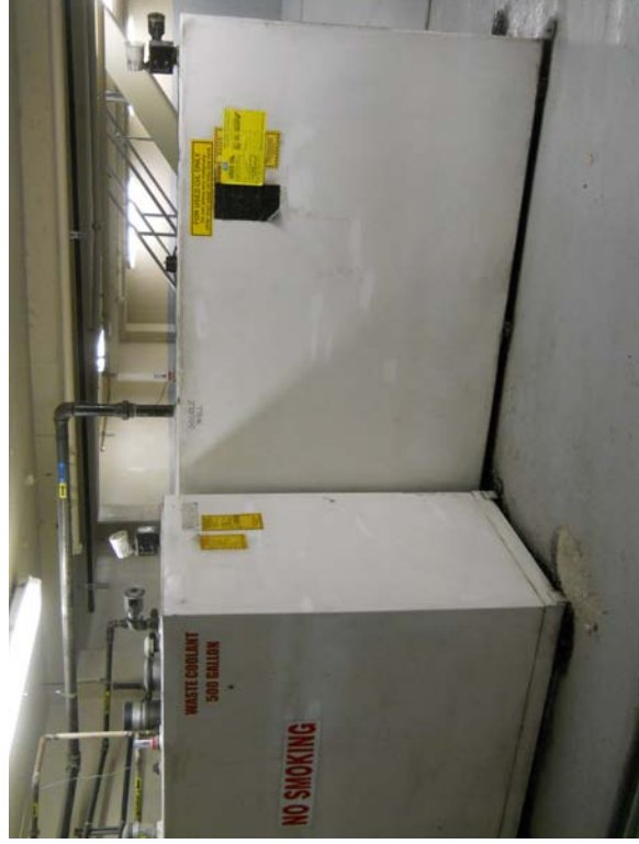
Figure 12 – Used Oil & Used Coolant ASTs in Basement
