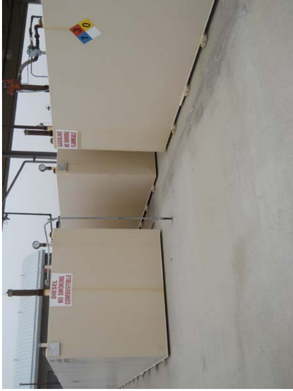
Figure 9 – Diesel and Gasoline ASTs @ Fuel Station
