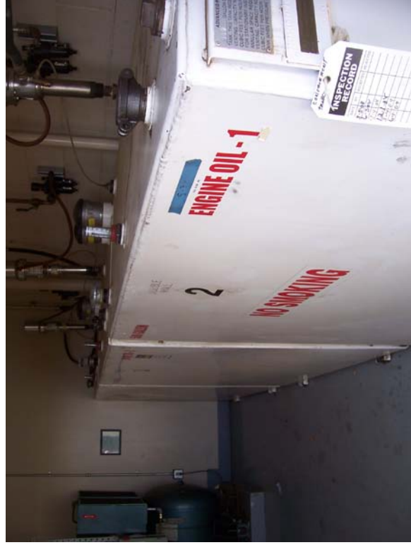
Figure 11 – ASTs inside Fuel Station Storage Room
